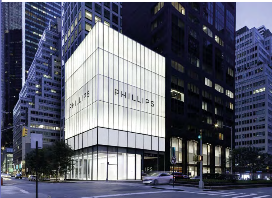
SEDE DA PHILLIPS / PHILLIPS' HEADQUARTERS
